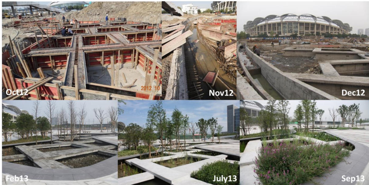
Figure 7 Collection of construction photographs
