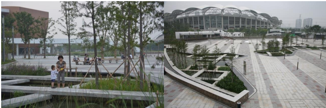
Figure 1 completed constructed wetlands
